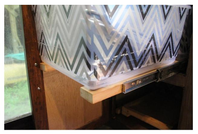
I used strips of wood attached to the floor of the cabinet to attach the drawer slide to. They were attached to the floor with metal angles. I used screws along with 3M VHB tape for the top since the shelf there is just thin paneling.
