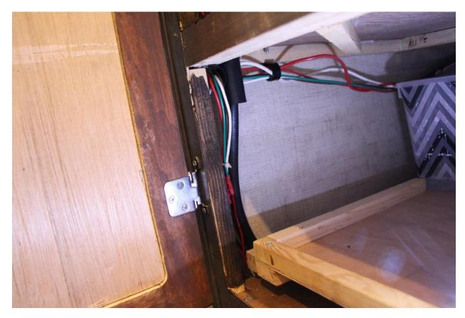
The drawers are composed of a couple of bins attached to strips of wood. I used ¾ X 1 ½ X 32 for the top and ¾ X 1 ½ X 25 for the bottom. The bottom is shorter than the top in order to accommodate the baffle that protects the Zamp plug and the tail light in the back of the cabinet.
