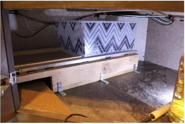
I used 26" drawer slides for the top and 24" slides for the bottom.
